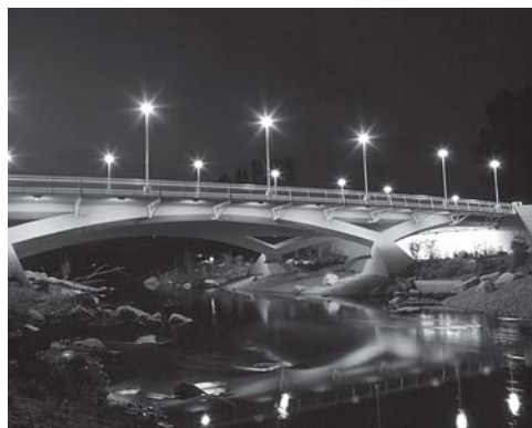
Above: NE 90th Street Bridge in Redmond, WA. New lighting credit criteria for LEED projects would create significantly challenge nighttime lighting on projects such as this urban bridge.
