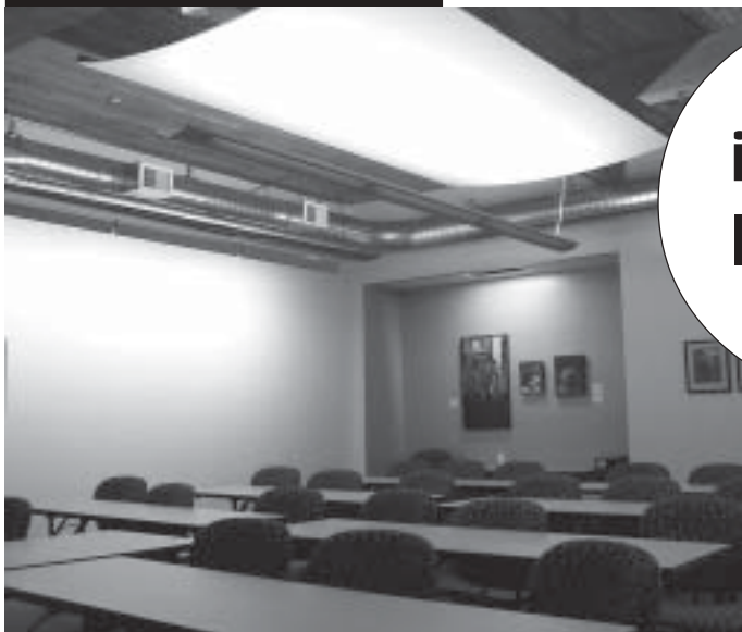
Above: The lighting in the meeting room at the Lighting Design Lab is almost completely indirect, using T5HO lamps.
