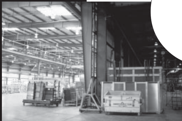
Northwest Industries Retrofit. Daylighting & Electric Light • photography, Barbara Erwine
